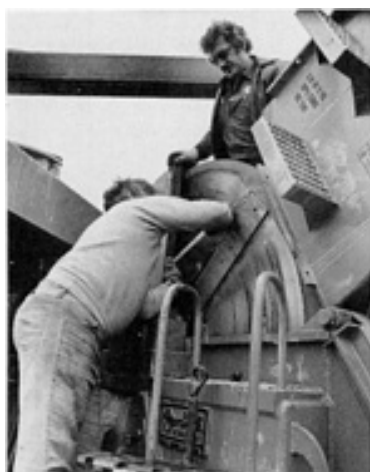
Fig. 7 Chipper knife being installed in a 75 in. Morbark total tree harvester
